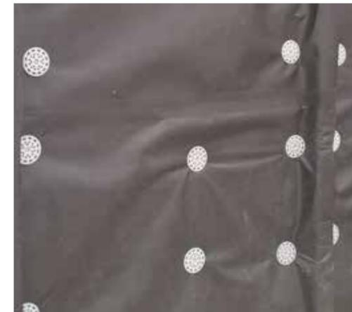
If an external airtightness line is required, plastic insulation anchors should be covered over with single-sided tape
