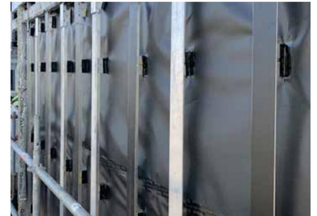
Tyvek® UV Façade Tape is a dedicated sealing tape suitable for sealing laps and bracket penetrations through Tyvek® UV Façade membrane
