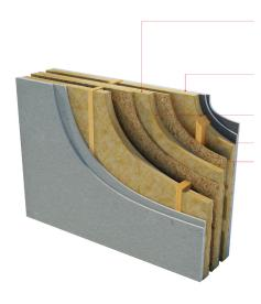
Wall width: 240mm (min) between inner faces of wall linings 50mm (min) cavity (gap between wall panels) 68mm (min) between stud frames
