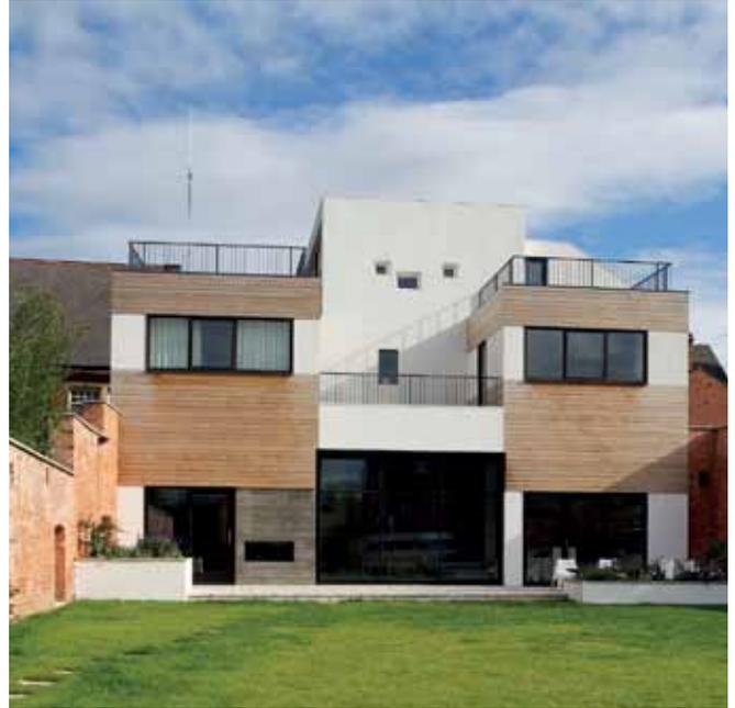
The new design involved demolishing most of the rear of the building but, where existing walls were retained, Aquapanel Exterior enabled the builders to improve the building's thermal performance to modern standards without making its footprint substantially bigger.
