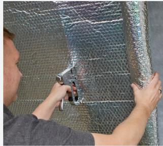
**4.** Tape and seal the perimeter and overlaps using YBS Aluminium Foil Tape, creating an airtight vapour control barrier.
